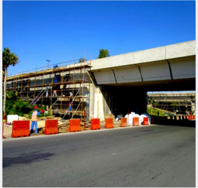
Bridge Structural Rehabilitation
