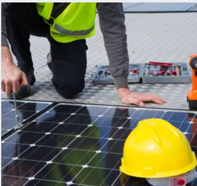
Solar Systems Installation
