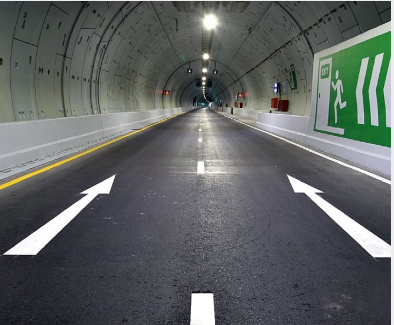
Tunneling from Ismailia Road Tunnels
