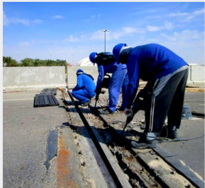
Expansion Joints Replacement
