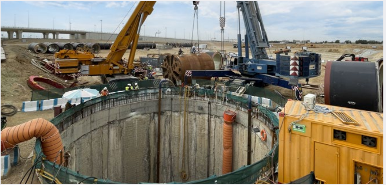
NWC Micro - Tunnel 3500 mm - Jeddah
