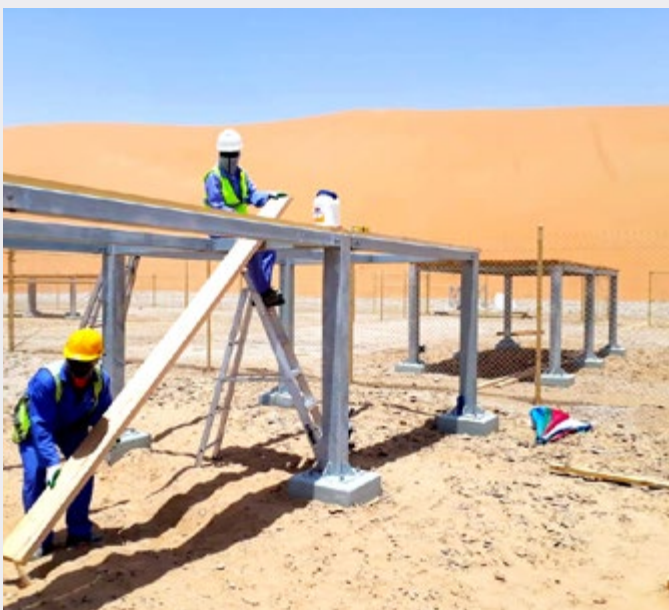
General Construction Work
