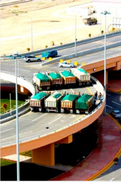
Bridge Load Test
